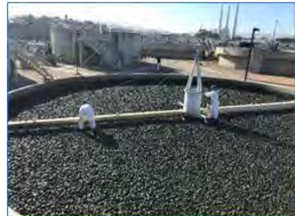
Staff performing trickling filter maintenance
