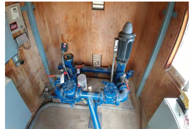
Elena Booster Station Pump motor repair
