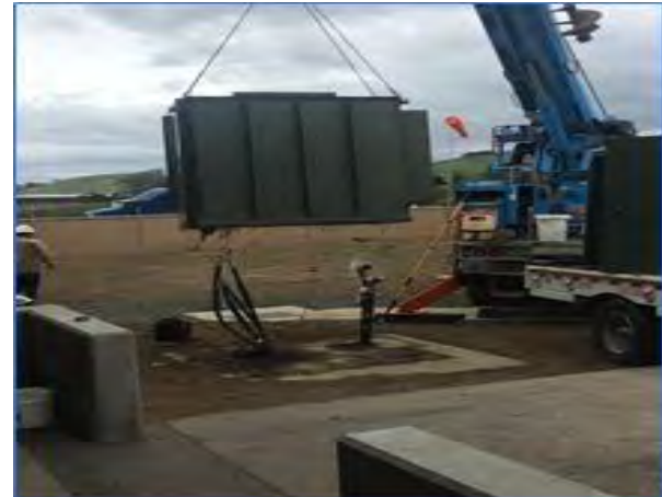
PG&E Transformer Replacement at the treatment Plant
