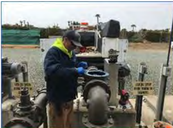
Check valve maintenance
