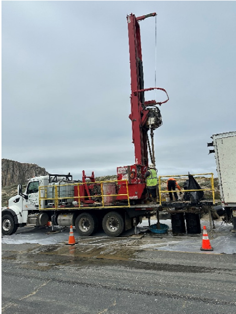
Well Site Coring – Sonic Boring #8 (SB #8)
