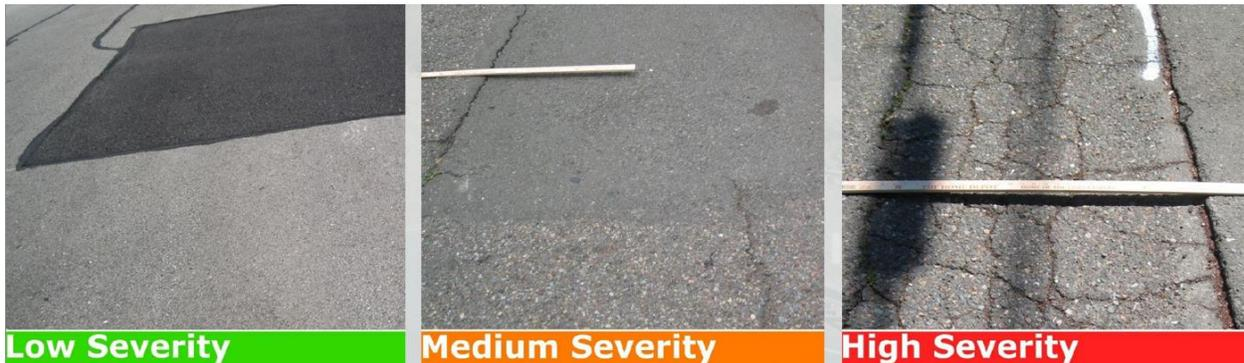
*Image 5: Patching and Utility Cut Patching*
