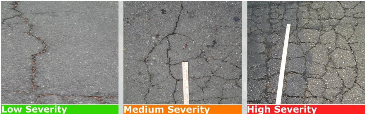
*Image 1: Alligator Cracking*
