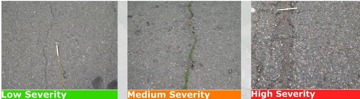
*Image 4: Longitudinal and Transverse Cracking*
